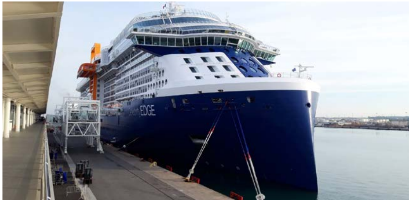
Figure 5: Ship Passenger Boarding Bridges ("Fingers")
